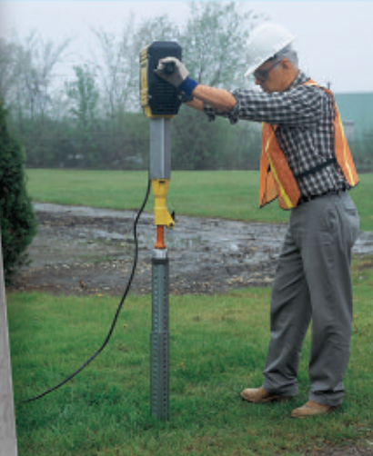
A minimum 30" piece of 12 gauge Telespar square steel tubing one size larger than the intended signpost is driven into the ground until 1-2 inches is left above the surface.
