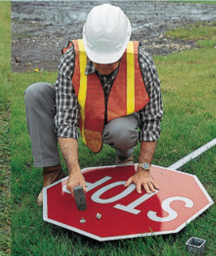
The sign is attached to a Qwik-Punch signpost, at ground level.
