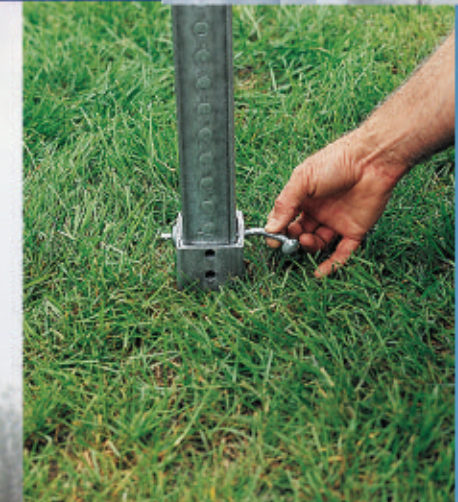
The signpost is secured to the anchor with a corner bolt or drive rivet.
