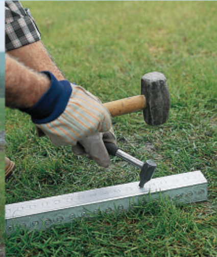
Die cut knockout is punched out of post at desired location.
